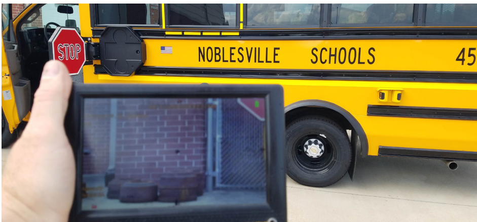
Noblesville School Bus, Stop Arm installation
